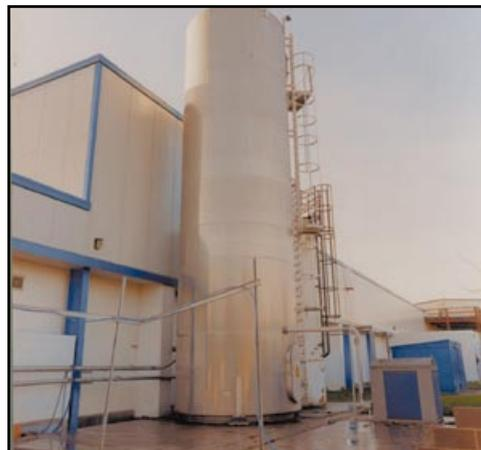
**Figure 58** Flour silos are confined spaces
