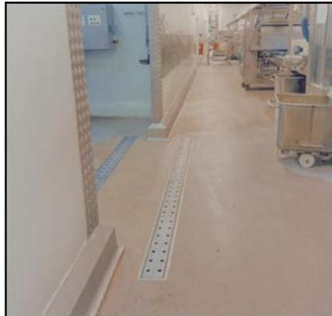
**Figure 29** Drainage channels for wet cleaning of floor
