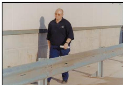
**Figure 32** Barrier to separate pedestrians from vehicles
