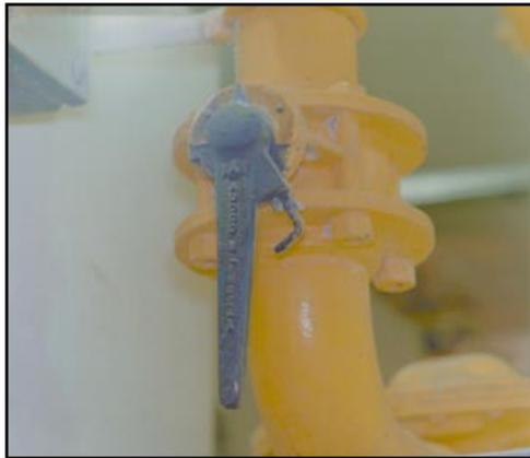
**Figure 73** Gas shut-off valve
