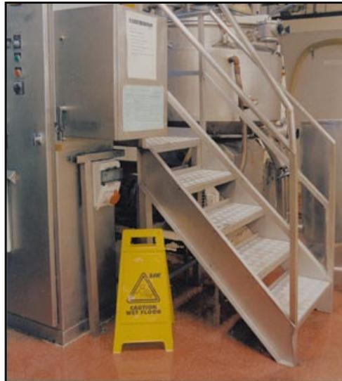
**Figure 44** Permanent-access stairs to plant with non-slip treads and handrails
