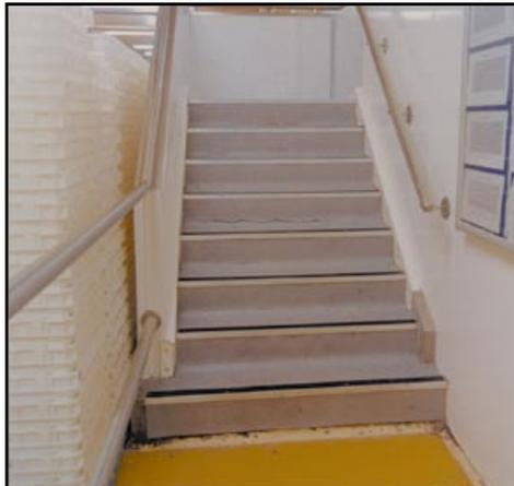
**Figure 45** Stairs with nosings and handrails
