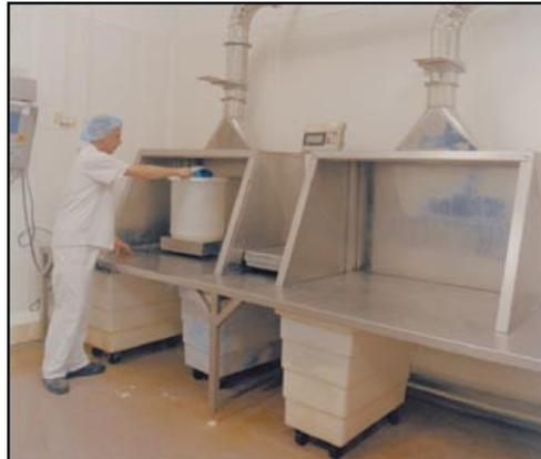
**Figure 19** Dust extraction at ingredients weighing station
