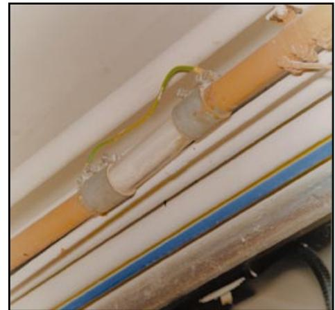
**Figure 66** Bonding connection between metal pipework on either side of viewpoint
