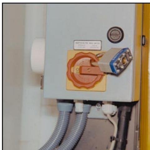
**Figure 51** Lockable isolator switch
